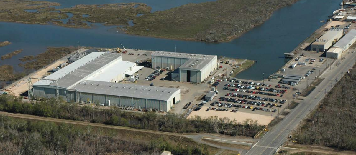
Textron Marine & Land Systems Manufacturing Facility, New Orleans, LA
